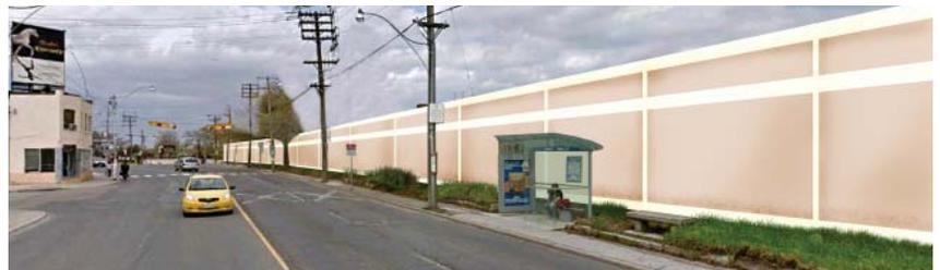
Brown & Storey’s rendering of Dundas Street West along the rail corridor with a 16-foot high concrete noise barrier. Metrolinx says that the rendering is not accurate and designs have not been finalized.
